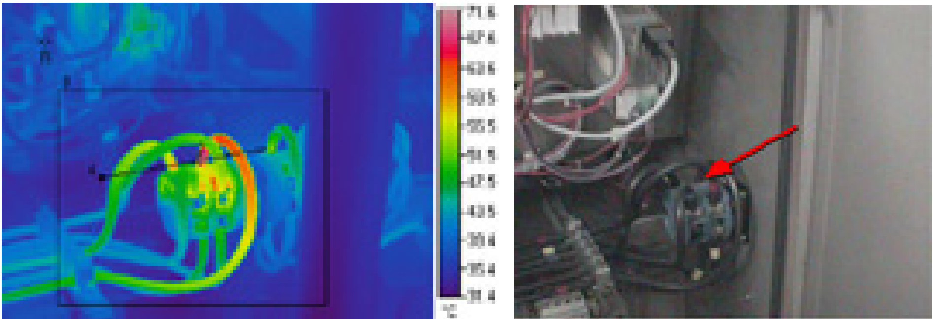
Images show poor connection on Main Isolator Switch
